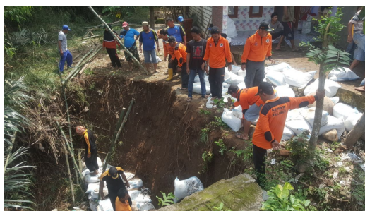
Figure 7. Structural mitigation after the flood disaster in Mojowarno District, 2022.
