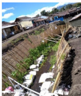
Figure 3. Embankments to protect the villagers' house
