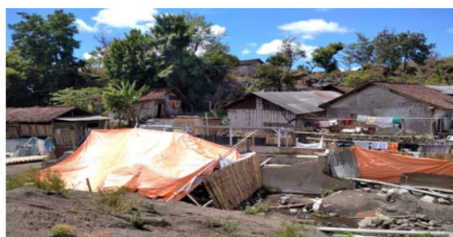
Figure 4. The repair process of houses and toilets
