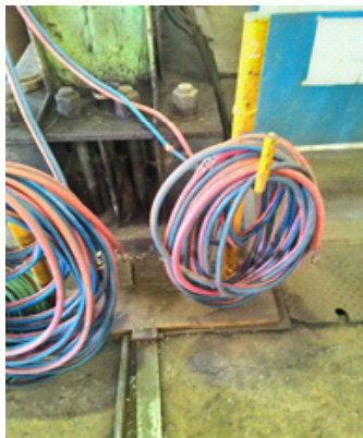
Figure 2. Cable Placement at Amurea II Plant III of Petrochemical Company in 2017
