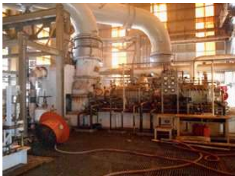
Figure 2. Work Area Situation in February 2019
