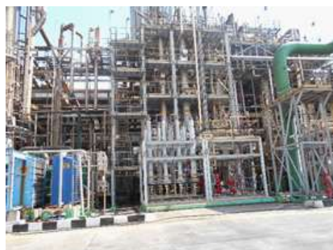
Figure 1. IA Ammonia plant of PT X Situation in February 2019
