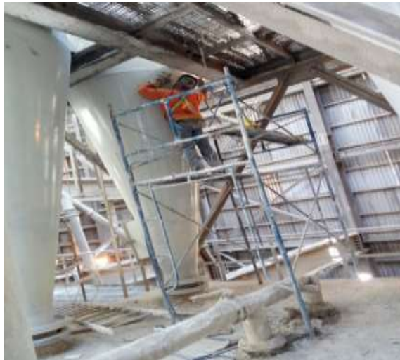
Figure 2. Welding Support Roller at a Gresik Fertilizer Company in 2017
