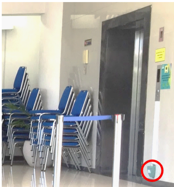
Figure 8. Modification pedal on the lift in the Rectorate Building of Universitas Airlangga in 2020
