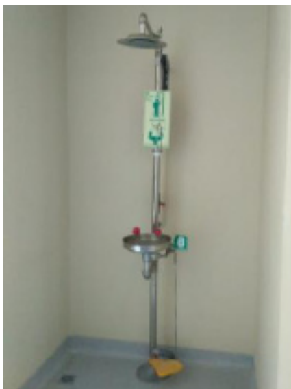
Figure 6. Condition of an Eyewash and Safety Shower at the Chemical Analytics Laboratory of University X Surabaya in August 2020
