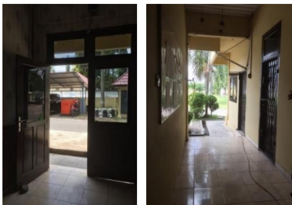
Figure 1. Main Door Corridor for Exit Facilities at Ogan Ilir Police Station
