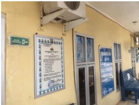
Figure 2. Directions of the Exit at Ogan Ilir Police Station
