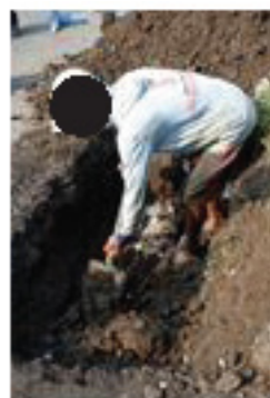
Figure 1. Excavation of Soil
