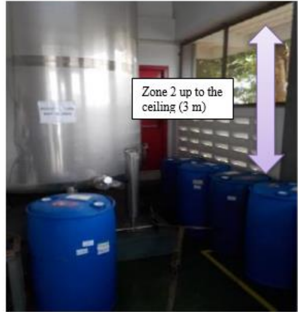
Figure 6. Zone for Ethanol Storage with Ventilated Wall
