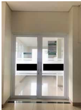
Figure 2. Gate of Bridge between Building A and B
