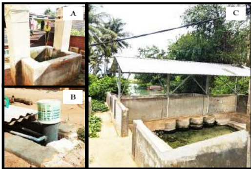
Figure 4. The non-piped water types are A) an open well, B) an artesian well, and C) a pond with outfall.
