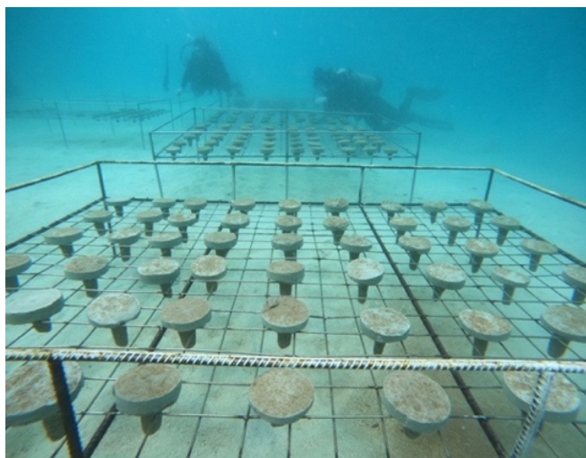
Figure 3. Design of coral table with iron frame model and cement media with sand mixture used for attachment of coral sampling fragments.
