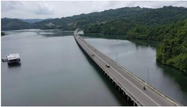
Figure 2. Aerial Photo of the 3.2 km Jayapura Ring Road
