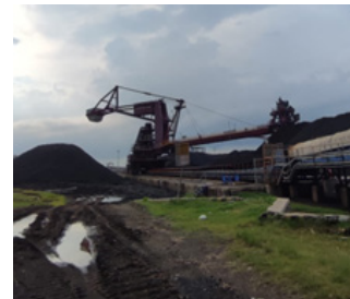
Figure 2. Stacker reclaimer PT. POMI
