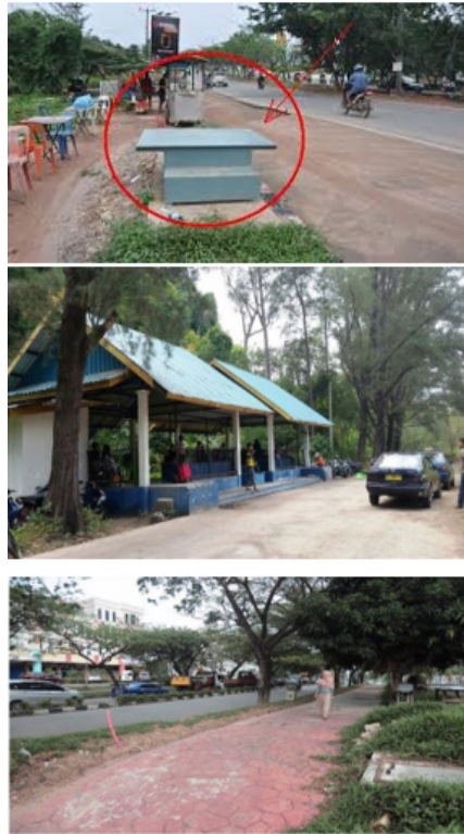
Figure 3. Condition of the Batam City bus stop Source: Dodo (2022)
