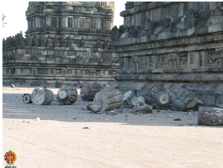
Figure 1. The Damage of Prambanan Temple caused by Earthquake on May 27 th , 2006 (sources: Dinas Perpustakaan dan Arsip Daerah Daerah Istimewa Yogyakarta )
