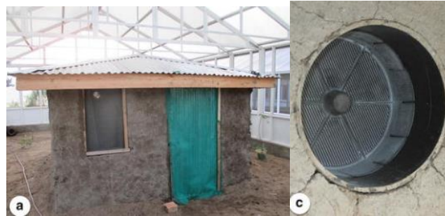
Figure 7. a. Experimental House With Mud Walls and Corrugated Iron Sheets Roof with Nets Inside, c. Eave Tubes Sideline with Insecticides (Deltamethrin and Bendiocarb) [41].
